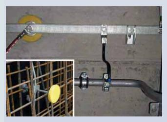
Fixed earthing terminals as corrosion-free connection
