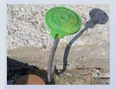
Protective cap to be attached to wires or strips as striking marker and accident prevention during the construction phase
