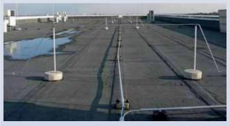
Elevated air-termination system with spacers and concrete bases in the range of the electrical installation on the roof
