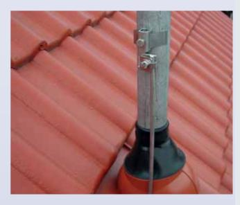
Pipe clamps for lightning current carrying capable connection e.g. of antenna poles and for lightning equipotential bonding according to EN 62305-3
