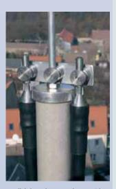
Parallel ducted HVI conductor with terminal clamp Part No. 301 329
