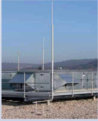
Isolated air-termination system for recooling plant with HVI conductor grey in a supporting tube
