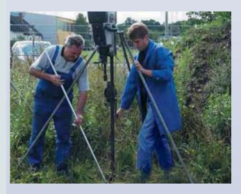
Hammer frame for driving of earth rods with a length of 1000 mm and 1500 mm with vibration hammer
