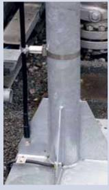
Connection of the HVI conductor at the earthing terminal
