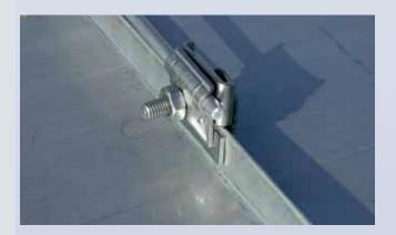
Clamps for connecting conductors to flanges of the same or other materials  $% \left( 1\right) =\left( 1\right) \left( 1\right)$
