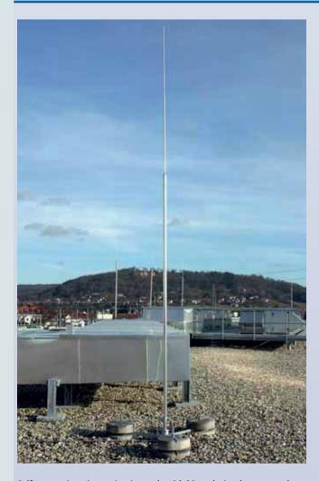
Self-supporting air-termination rods with hinged tripod to protect larger roof superstructures and adjustment to the roof pitch up to max.  $10^\circ$  The air-termination rods are dimensioned for wind velocities up to 145 km/h (wind load zone II).
