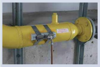
Pipe clamp for electrical contacting of pipes in explosion-hazard areas for implementing of lightning equipotential bonding according to EN 62305-3
