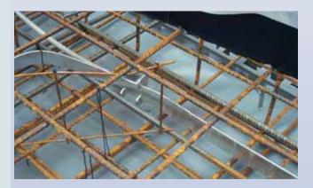
Clamps for connecting round and flat conductors in the concrete foundation
