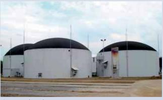
Biogas/natural gas plant Kerpen, Germany Protection of the fermenters – air-termination masts with HVI conductors
