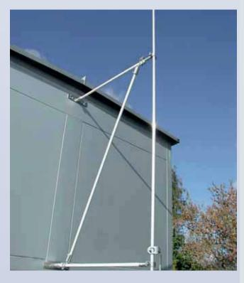
Variable range of supports for conductors and air-termination rods for keeping the separation distance according to EN 62305-3
