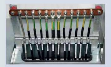
Equipotential busbars for the protective and functional equipotential bonding and lightning equipotential bonding according to EN 62305-3 also for use in potentially explosive atmospheres (screws are locked to prevent accidental loosening)
