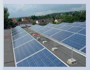
Spacer with concrete block and support plate, loose conductor leading
