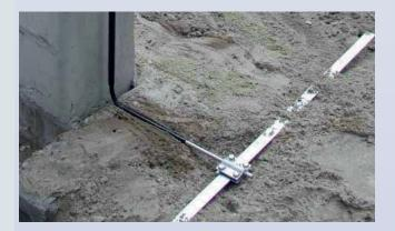
Cross units for aboveground and underground connection of conductors in cross arrangement and T arrangement
