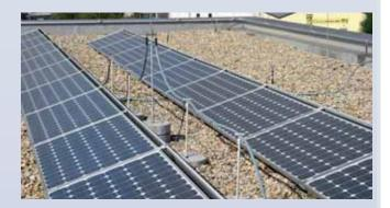
HVI conductor light is the system for keeping the separation distance on flat roofs. Uncontrolled flashover e.g. through the roofing to metal or electrical parts underneath will be avoided by the high-voltage resistant insulation of the HVI conductor light.
