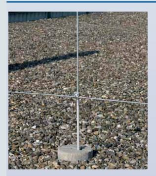
Air-termination rods for the implementation of isolated air-termination systems e.g. on flat roofs, installed on wedge mounting contrete base
