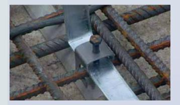
Clamps for connecting concrete steel mats or reinforcements with round and flat conductors
