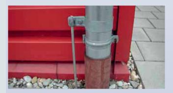
Pipe clamps for lightning equipotential bonding connection of downpipes according to EN 62305-3
