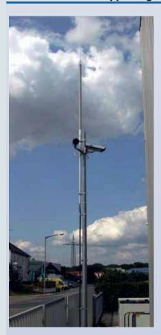
HVI conductor inside of the supporting tube, optically adjusted, provides little wind exposed surface
