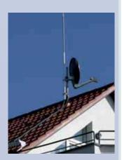
Detail – supporting tube with installed conductor
