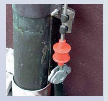
TFS: High-capacity isolating spark gap
