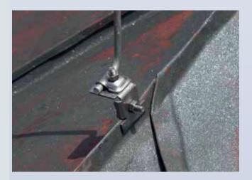
Clamps for connecting conductors with seams enlarged contact surface
