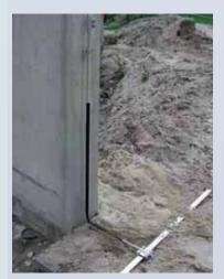
Earth entry rods for connecting the down conductors to the earth-termination system
