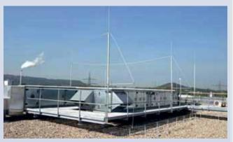
Isolated air-termination system DEHNiso Combi
