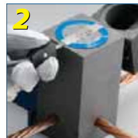
2 Attach control unit termination clip to ignition strip
