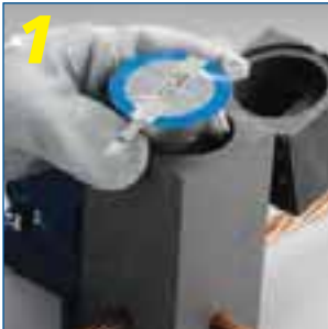
1 Insert CADWELD® PLUS package into mould
