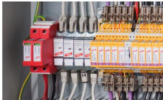
Figure 11 Example of surge protective devices in a pitch system
