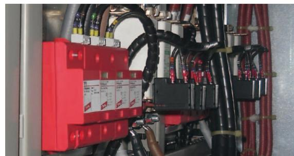
Figure 8 Protection of the rotor winding of the generator ("Neptune" circuit)
