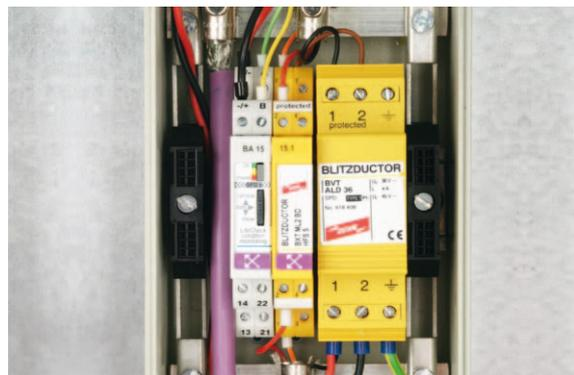
Figure 10 Protection of the weather station (anemometer)
