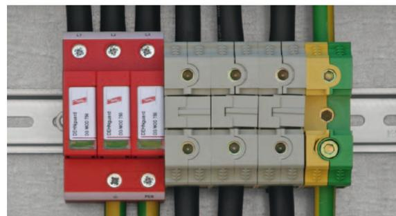
Figure 9 Protection of the stator side of the generator
