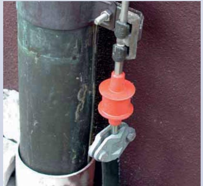
**TFS:** High-capacity isolating spark gap
