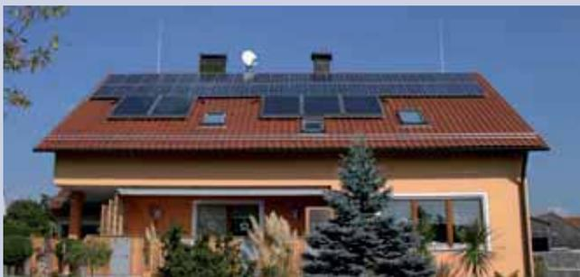
Isolated air-termination system – all roof-mounted structures such as solar thermal, PV and exhaust systems incl. the parabolic antenna in the protective area
