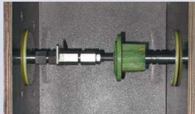
Figure 1: Wall bushing with formwork installation
