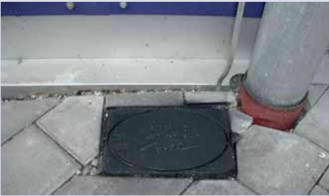
Test joint boxes for underfloor mounting to disconnect the down conductor from the earth-termination system for measuring purposes
