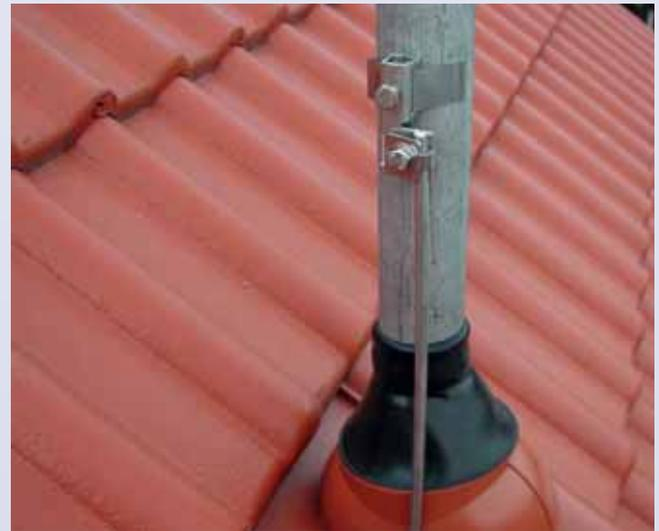
Pipe clamps for lightning current carrying capable connection e.g. of antenna poles and for lightning equipotential bonding according to EN 62305-3
