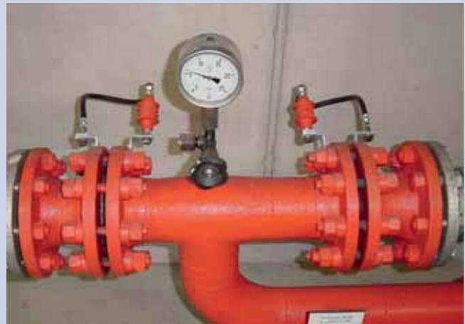
The Ex isolating spark gaps of the EXFS 100 / EXFS 100 KU product family are used when conductive installation components situated in explosion-hazard areas cannot be connected directly with each other. The spark gaps with low sparkover voltage are especially efficient for isolated installation components with little insulation resistance. No special regulations have to be observed for safe application in zone 1 with gases or zone 21 with dusts.
