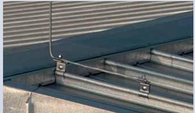
**for roofing with round standing seam, with clamping frame**
