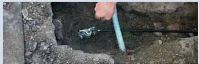
Brackets for connecting round conductors, cables and flat strips to earth rods
