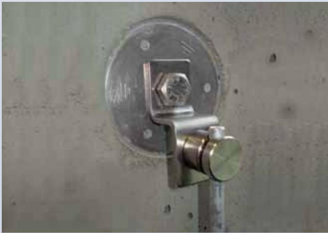
End pieces for screwing on the fixed earthing terminal (FET) for connecting e.g. an equipotential bonding bar or for connecting construction elements (e.g. steel girders or alike) by screwing or welding
