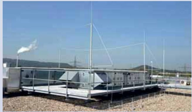
Isolated air-termination system DEHNiso Combi
