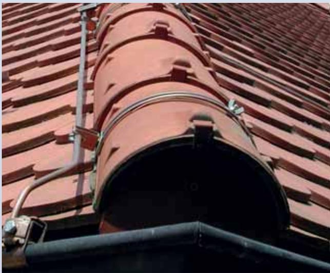
Conductor holder for air-termination conductors to be fixed at the ridge e.g. of tiled roofs
