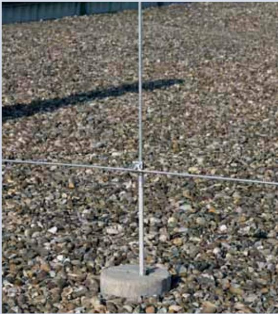
Air-termination rods for the implementation of isolated air-termination systems e.g. on flat roofs, installed on wedge mounting concrete base
