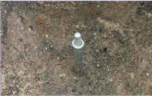
Earth rods for implementing earth-termination systems for down conductors or transformer stations
