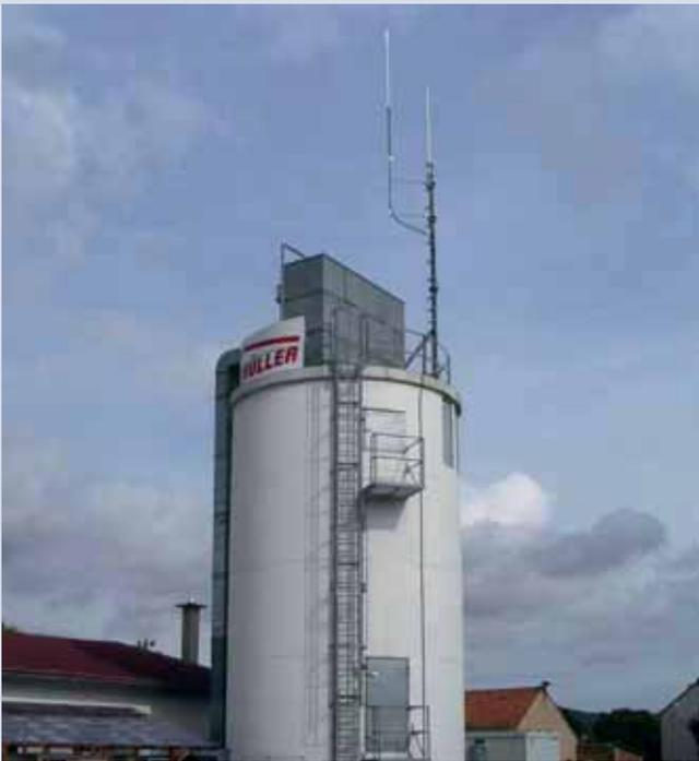
Antennas with a radiation characteristic of 360° are used in different fields of radio application. Such antennas are known as "omnidirectional antennas" on the market. Typical applications of omnidirectional antennas in practice are private mobile radio (PMR) systems, safety nets and sometimes also GSM networks. In GSM networks, however, they are only applied if there is a low frequency of radio waves.
