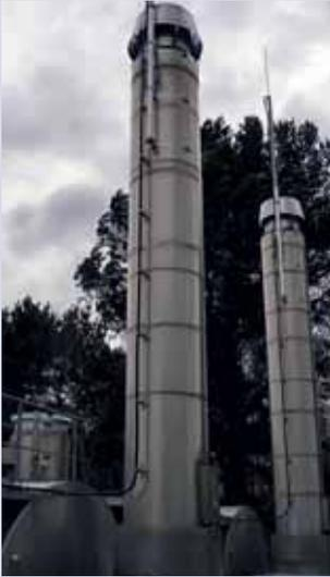
HVI conductor installed in Ex zone 2
