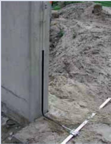
Earth entry rods for connecting the down conductors to the earth-termination system
