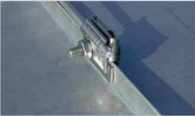
Clamps for connecting conductors to flanges of the same or other materials
