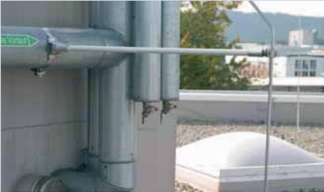
Spacer with attachment, fixing bush and tensioning strap
