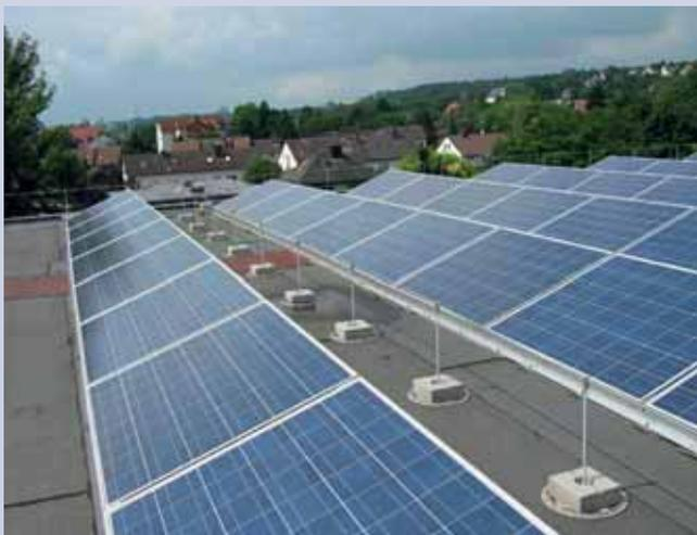
The roof conductor holders are dimensioned for wind velocities up to 145 km/h and 162 km/h (wind load zone II and III) provided that the specified distance  $\leq 1.2$  m is complied with.
