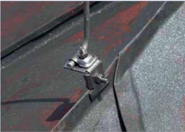
Clamps for connecting conductors with seams
