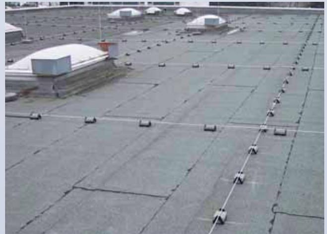
**double conductor retention Type FB2**
