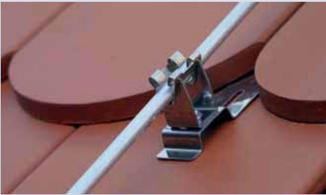
Roof conductor holders for fixing of air-termination conductors and down conductors
