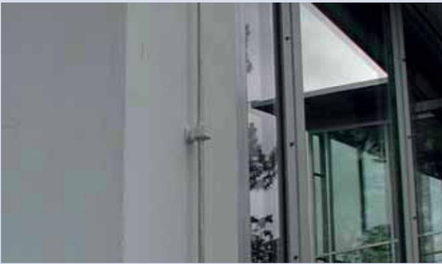
plastic holder system with loose conductor leading
