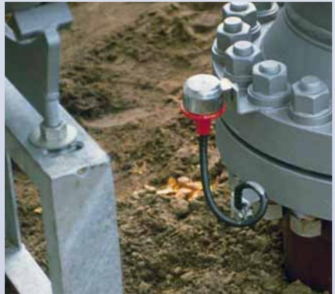
Ex isolating spark gaps of the EXFS L / EXFS KU product family are used when the direct interconnection of electrically conductive installation components in Ex areas is not applicable. As, for example, in case of cathodically corrosion protected pipeline sections.
