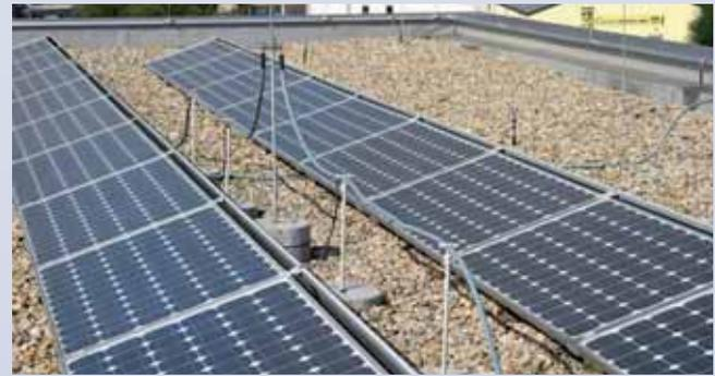
HVI conductor light also allows for installations without performing an equipotential bonding with the building or structure at the end of an adjustment range.
