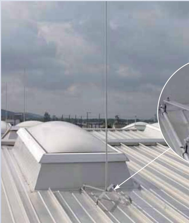
Air-termination rods for protecting roof-mounted structures, domelights etc. Brace ends (borings  $\varnothing 11$  mm) to be fixed by means of four roof conductor holders.
