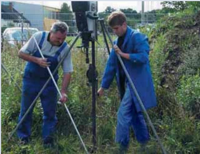
Hammer frame for driving of earth rods with a length of 1000 mm and 1500 mm with vibration hammer
