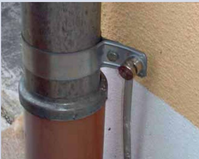
Clamping screw connector for lightning current carrying capable connection of round conductors e.g. to flat profiles, downpipe clamps or other parts of the lightning protection system
