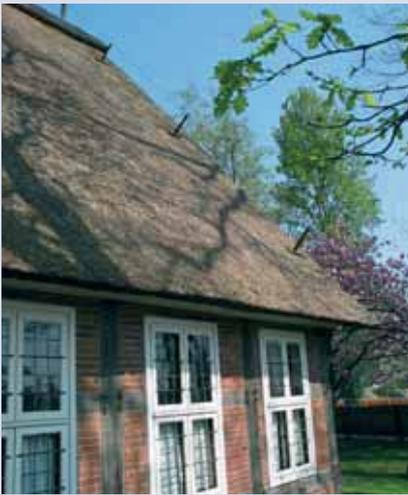
On thatched roofs the air-termination conductors have to be installed as elevated traverses e.g. on isolating supports. Certain distances have to be kept also to the eaves.
