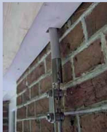
Figure 3: Connection to down conductor – bushing of cornice board
