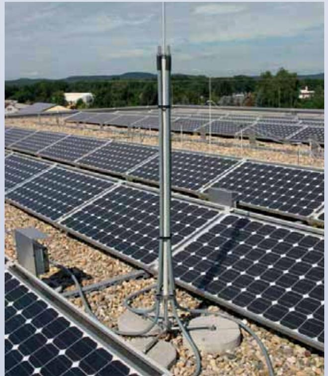
**Air-termination mast 30 for HVI conductor light SET I 2600 mm total height**
